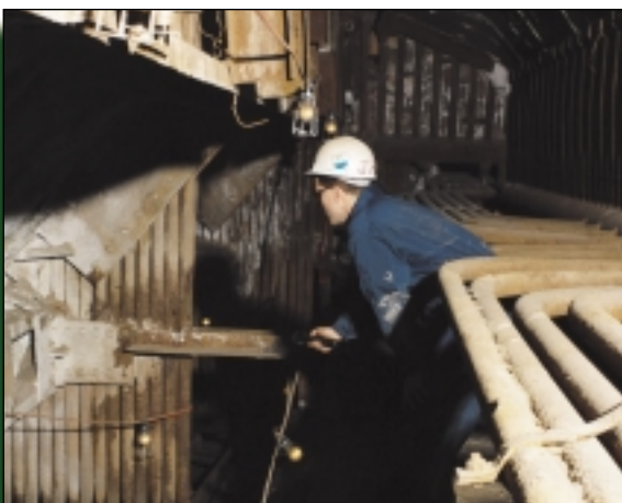
Figure 13: Boiler fitness surveys include a thorough inspection of your boiler to identify opportunities for improved performance.
