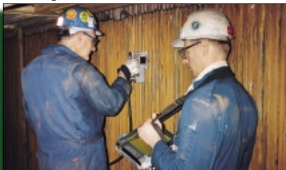
Figure 9: The exceptional testing speed of the FST-GAGE™ allows B&W technicians to scan thousands of feet of boiler tubing.
