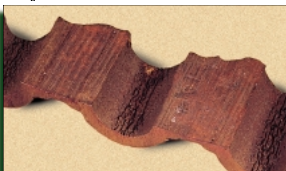
Figure 10: Corrosion fatigue cracks in membraned wall tubes.
