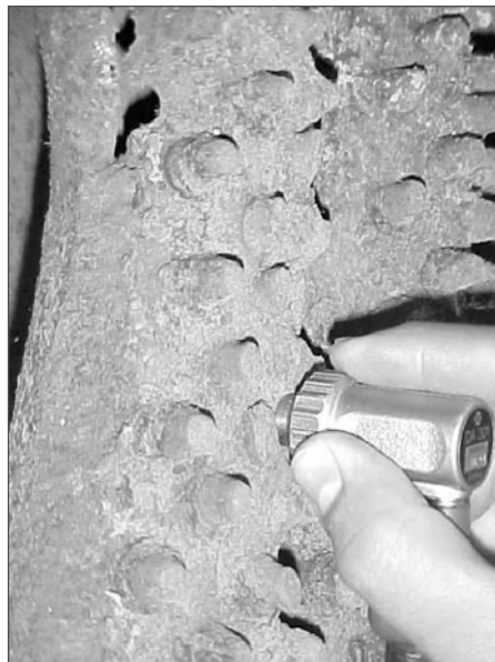
12. Ultrasonic thickness survey on a studded tube of a recovery furnace.
