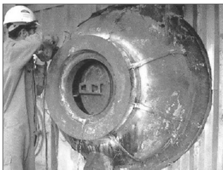
9. Non-destructive testing (magnetic particles) in progress in the water drum of a recovery boiler.
