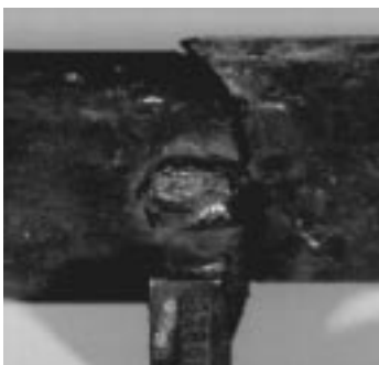
Mechanical fatigue failure at an attachment
